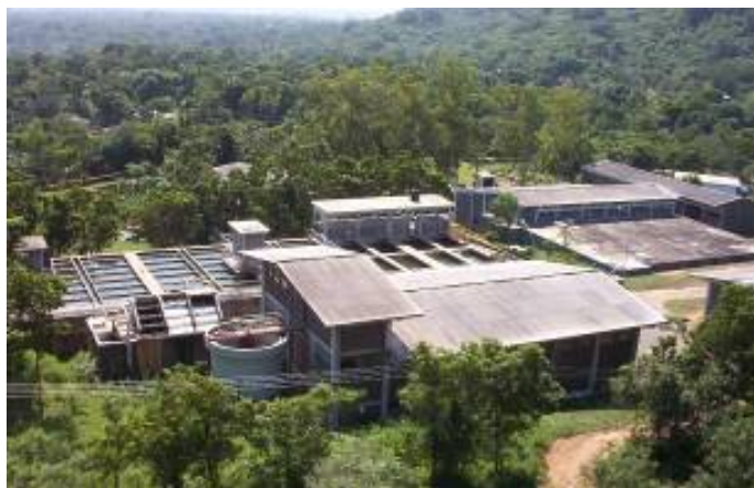
Kantale water supply plant in Trincomalee
